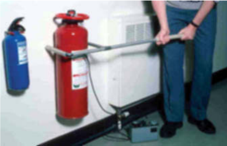
FIG. 6. Mobile gauge for detecting the level of liquids in closed fire extinguisher cylinders (courtesy: National Radiological Protection Board, UK).
