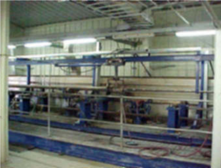
FIG. 37. Facility for tubular decontamination by HPWJ (courtesy: Atomic Energy Commission of Syria).
