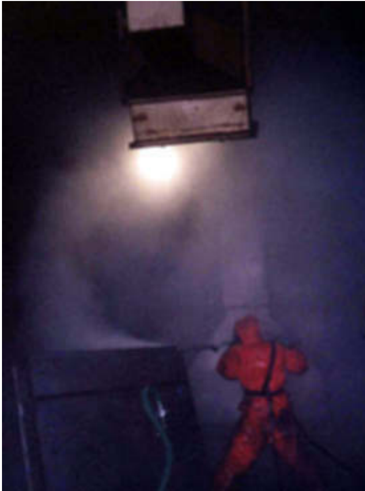
FIG. 36. Workers using HPWJ lance (overhead extractor removes airborne contamination) (courtesy: Atomic Energy Commission of Syria).
