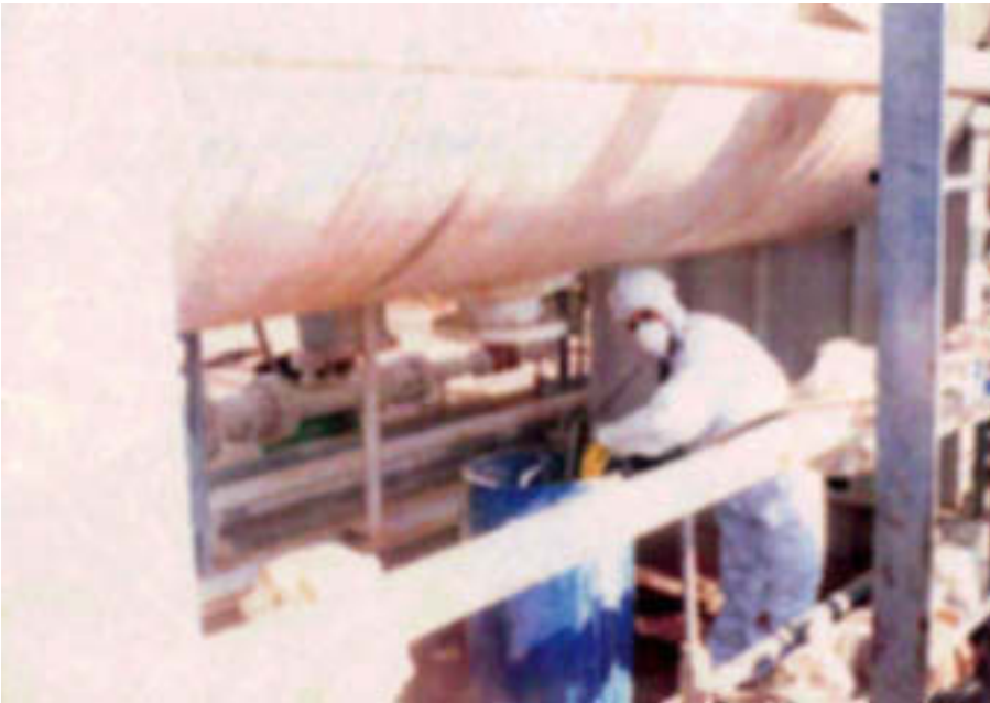
FIG. 34. Removal of bulk sludge from a vessel (courtesy: Atomic Energy Commission of Syria).
