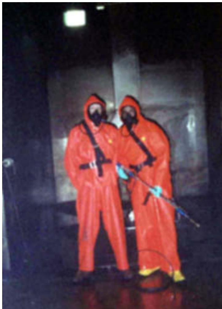
FIG. 35. Workers with personal protective equipment and HPWJ lance (courtesy: Atomic Energy Commission of Syria).
