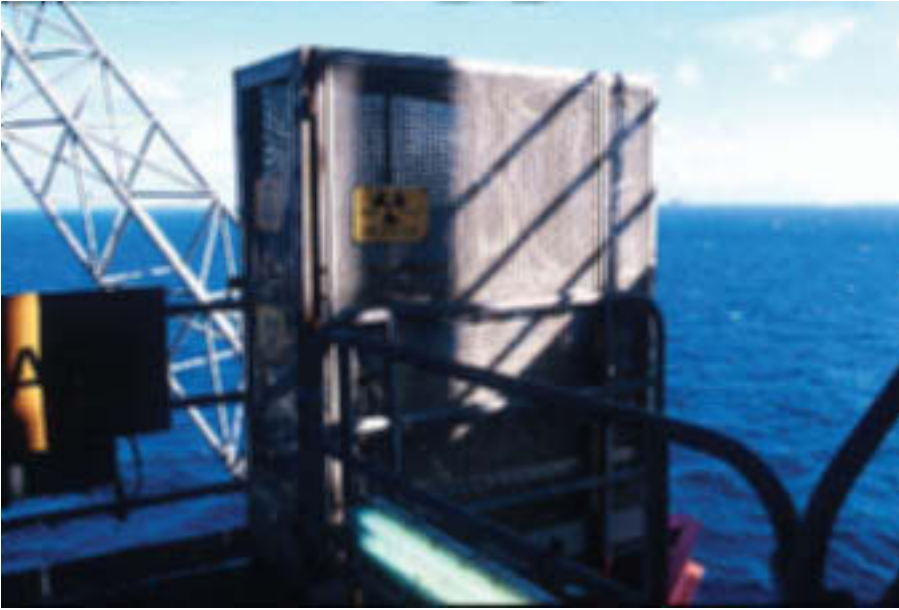
FIG. 16. Store for radioactive sources (courtesy: National Radiological Protection Board, UK).
