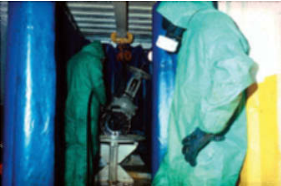
FIG. 26. Workers wearing personal protective equipment decontaminating a valve inside an on-site facility (courtesy: National Radiological Protection Board, UK).
